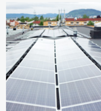
SOLAR PANELS INSTALLED AT NORWAY HEAD OFFICE
